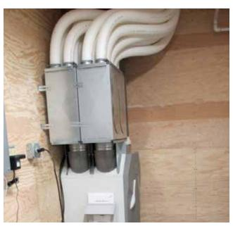
Energy-recovery ventilators (ERV's) bring fresh, outside air into your home and replace stale, polluted indoor air. ERV's also recover some of the heat and humidity from exhausted indoor air and add it to the cool, dry incoming air. This process is reversed in the warm months when indoor air is cooler and dryer than outside air.
